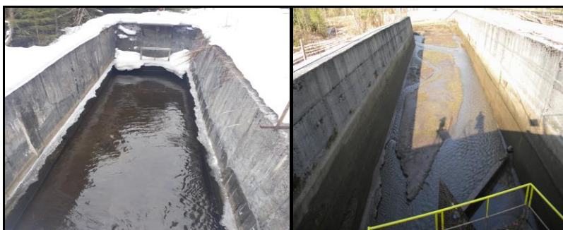
Figura 5.13 Bazinul deznisipator al CHEMP Vorova (original) Figure 5.13. De-sanding basin of Vorova SHP (original)
