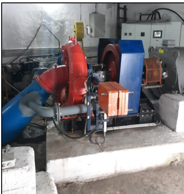
Figura 5.10 Turbina FO 90/570 din CHEMP Sihăstrie (original) Figure 5.10 FO 90/570 turbine of Sihastrie SHP (original)
