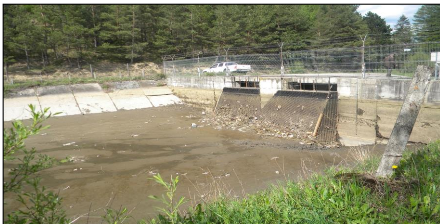
Figura 6.10 Bazin compensator colmatat CHEMP Pojorâta (original) Figure 6.10 Silted forebay tank at SHP Pojorata (original)
