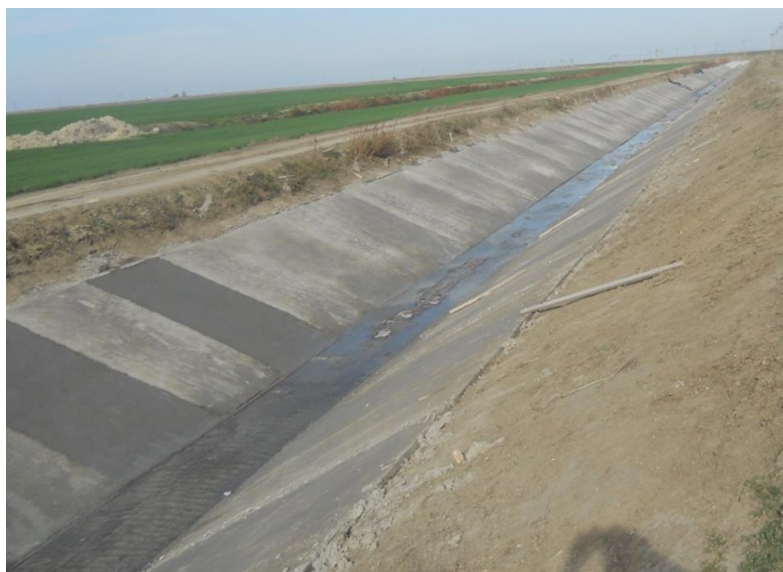
Figura 5.13 Rostuire pereu Figure 5.13 Sealing the joints
