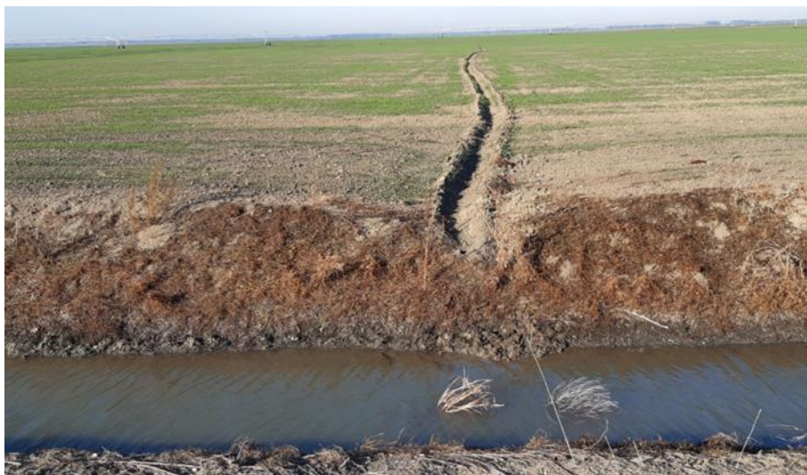
Figura 5.4 Canal secundar de desecare Figure 5.4 Secondary drainage channel
