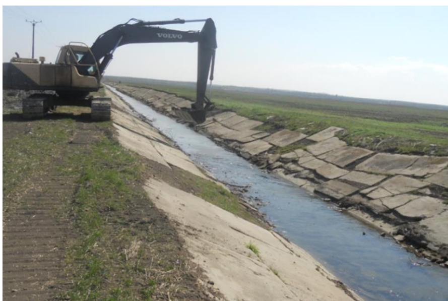
Figura 5.11 Degajarea dalelor sparte Figure 5.11 Removing broken tiles
