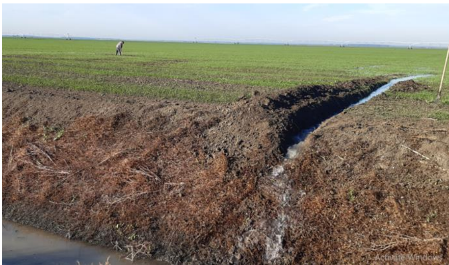
Figura 5.2 Canal colector Figure 5.2 Collector channel
