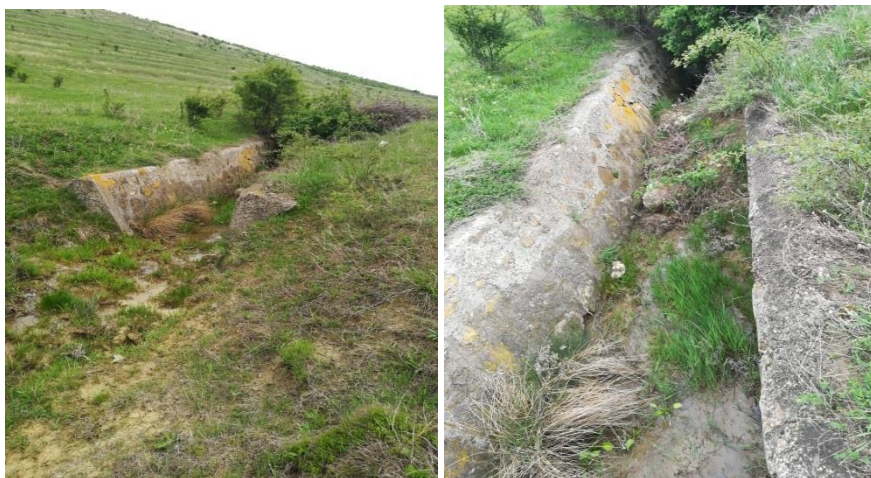
Figura 6.16 Debușeu din beton colmatat pe pășune, Deleni (original) Figure 6.16 Concrete outlet filled on pasture, Deleni (original)
