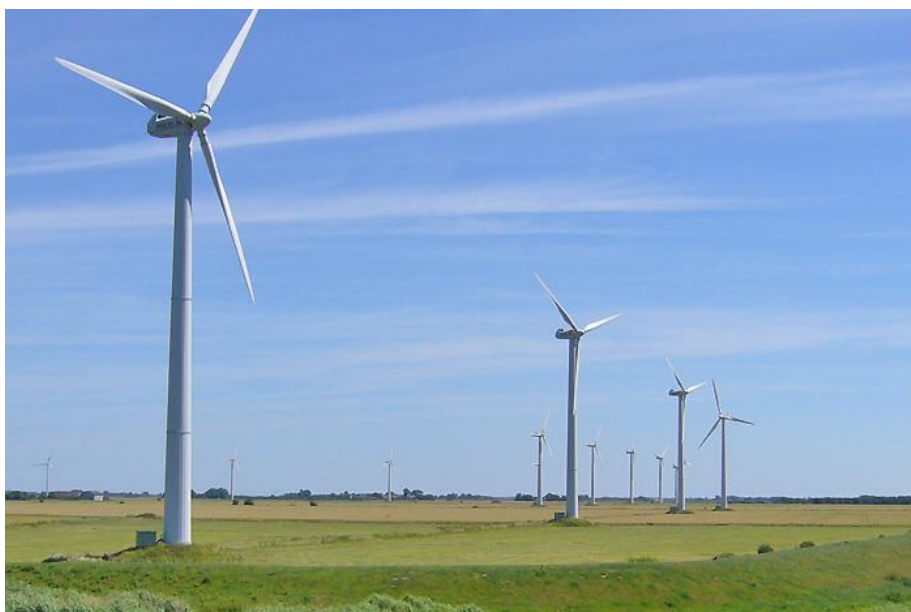
Fig. 4.13 Turbine eoliene instalate de SC Energopark SRL
